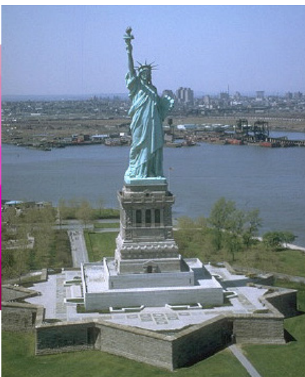
1884 Dyckerhoff supplies 8,000 wooden barrels of cement for the foundation of the Statue of Liberty in New York
